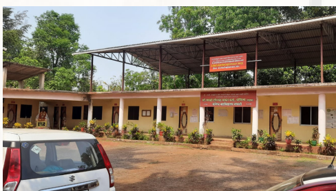
CONSTRUCTION OF ENTIRE 1ST FLOOR AT KANISHT MAHAVIDYALAYA, NAYASHI, CHIPLUN
